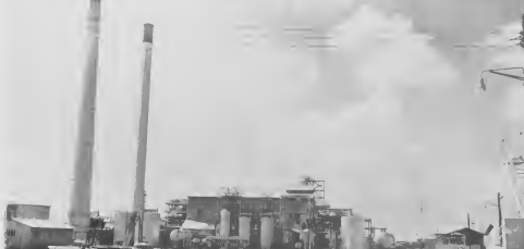
VERTICAL APPLICATION of No. 3 Edeleanu Plant conserves space as opposed to horizontal application of the original Edeleanu installations, built in 1938.
